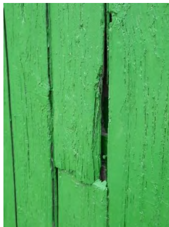
Plate 4.17: Broken Garage Door Panel
